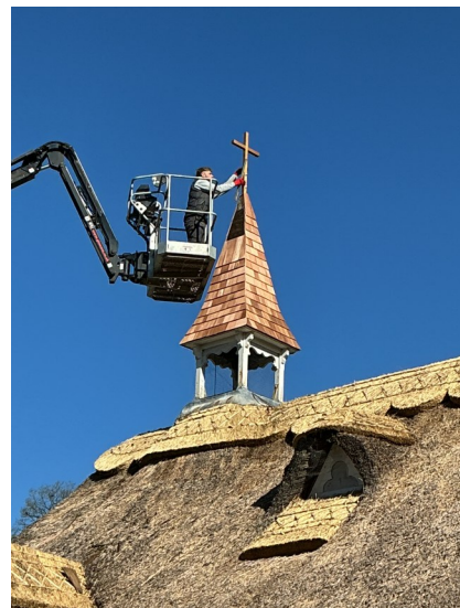
Repairs to All Saints roof took place this week
